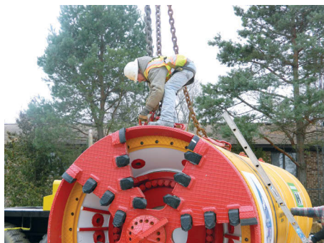
LEFT: The TBM being lowered into the pit to begin excavation. (Photo provided)
