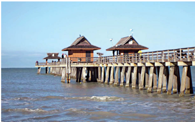
Repairs to the Naples, Fla., public pier had been previously postponed. With the state better able to take care of itself now, property taxes have been made available for this and similar projects. The pier structure suffers from a high percentage of severe corrosion, and in some cases, total obliteration of connection hardware. (Photo provided)
